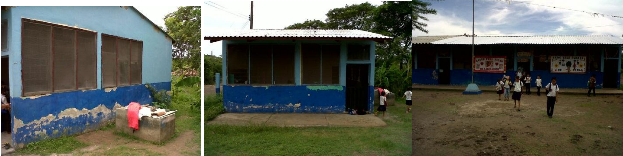
Side of school Kindergarten
